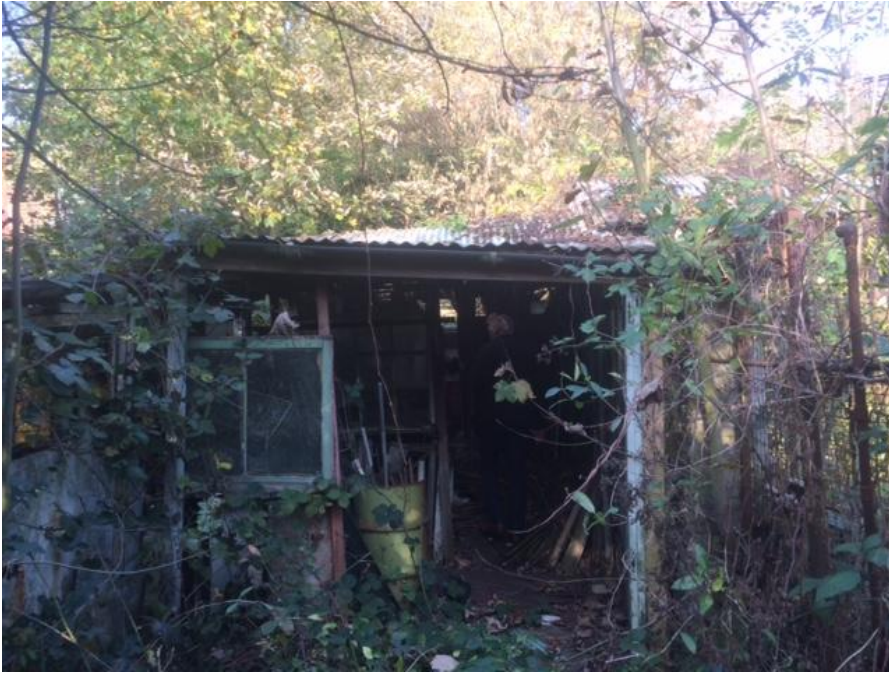
Site visit photo - existing structure on site (looking west)
