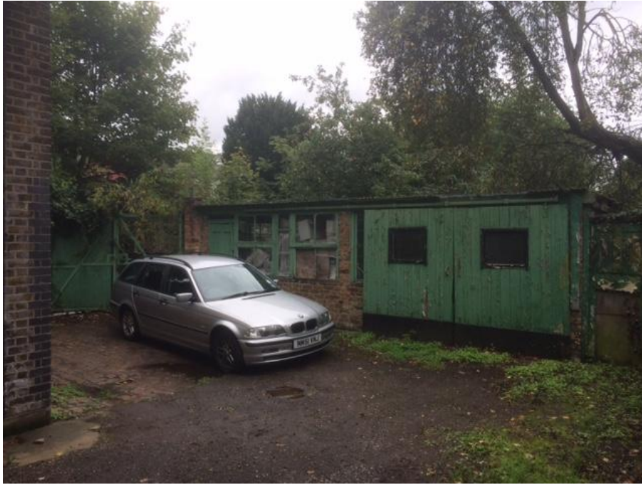
Site visit photo – existing garage building
